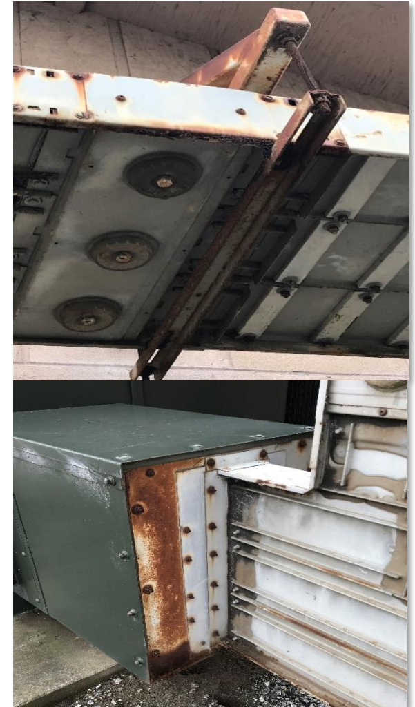
Significant Corrosion (Transformer Busway)
