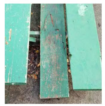
• The wood bleacher systems at the softball field are extremely weathered with much of the paint having pealed away and some sections having broken and split off.
