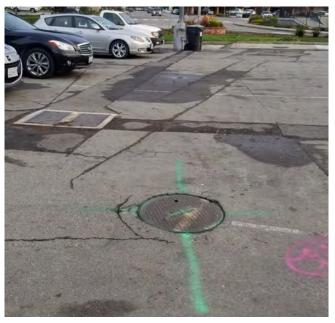
Most of the northern parking lot along main street is covered in cracks and patches due to years of use and numerous trenching operations. All northern parking lot asphalt has a very weathered appearance.
