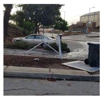
The pipe gate that serves as the barrier for the access road up to the hilltop area from the southern parking lot has been bent and no longer can be shut and locked.
