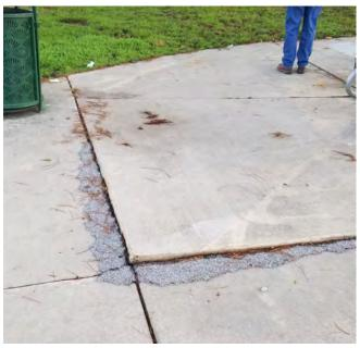
Concrete paving is lifting in areas around the park creating tripping hazards. City maintenance has patched some of these areas of lifted concrete with a slurry mix that creates a temporary and patchy appearance.
