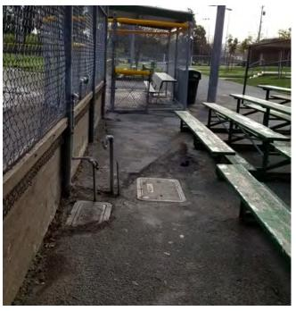
An old drinking fountain has been removed from the spectator area behind the softball backstop, but the exposed piping has been left above grade creating a potential tripping and safety hazard.
