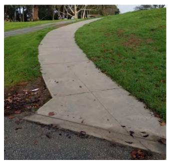
The pathways that lead up to the hilltop site amenities have a slope that is greater than 5%, and are out of ADA conformance.
