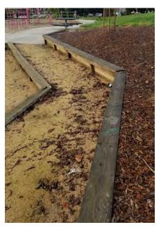
The wood at the terraced amphitheater area is leaning and lifting from the retained grades behind it, and some of the wood is starting to rot.
