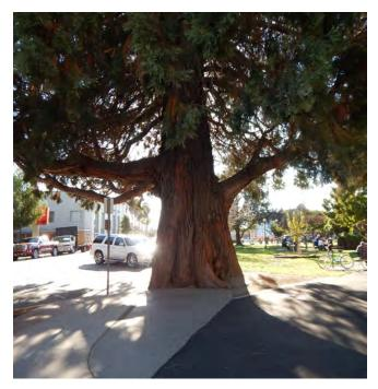
• The large giant sequoia's roots are lifting the concrete and asphalt at the corner of Peck Street and Union Street.
