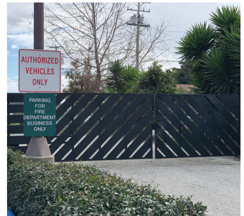
The new gate at Fire Station 1 keeping watch over the equipment.
