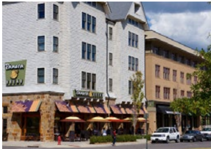
Heavy stone used below lighter siding material.
