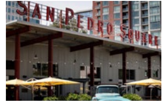
Projecting Roof Eave
