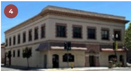
4 Porter Building 280 Main Street
