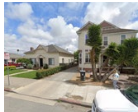
VEHICULAR DRIVE INTO A LOT —Vehicular drives are to be located and designed so as to preserve the beauty and function of a walkable Downtown environment. See Standard 6.5.A.3.b.
