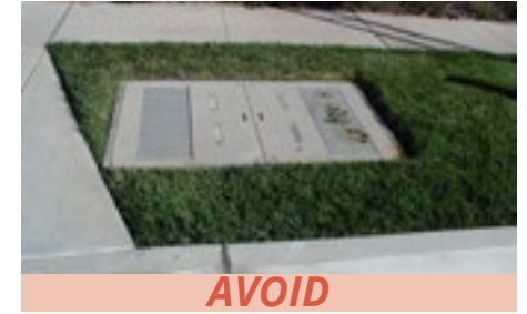
Example of inappropriately placed ground-level utilities in a parkway.
