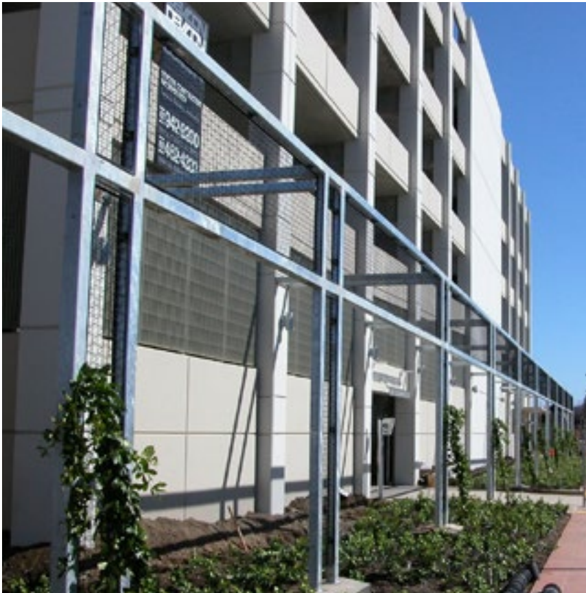
PHOTO CAPTION —Watsonville Civic Center Parking Structure
