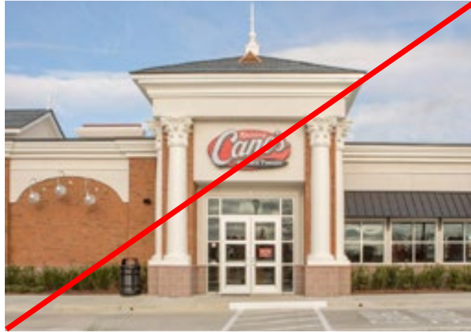
Fiberglass classical ornamentation and poorly applied.
