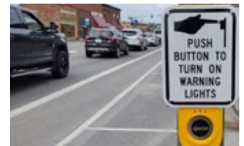
TOP TO BOTTOM —Example of a high-visibility crosswalk and pedestrian activated warning system
