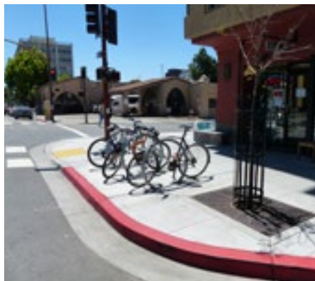
TOP TO BOTTOM —Example of a wide, unobstructed sidewalk with pedestrian amenities and curb bulb-out
