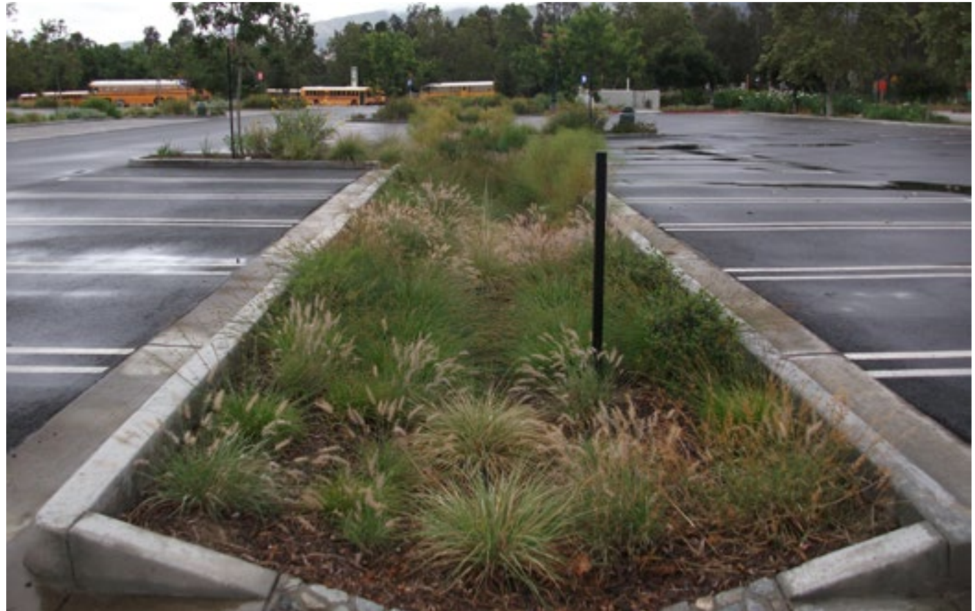
PHOTO CAPTION —Bioretention filter
