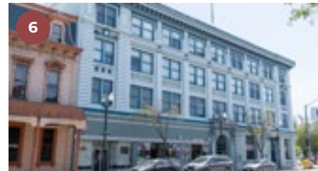
6 Lettunich Building 406 Main Street
