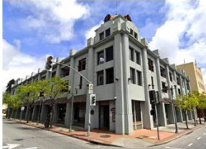
The façade of the existing parking structure at the corner of Beach and Rodriguez Streets in Downtown Watsonville is organized like a typical Downtown building and the ground floor is lined with occupiable space.
