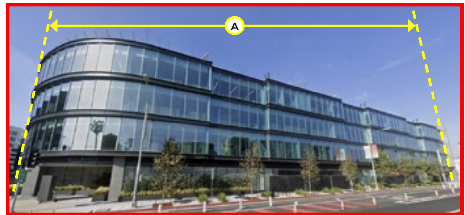
AVOID: This façade would feel inappropriately massive and monotonous in Downtown Watsonville. Façades whose overall length (A) exceeds that listed under Applicability in Table 6-6 need to be broken into multiple Massing Increments.
