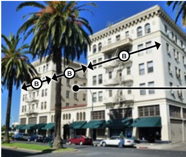
UPPER-LEVEL FORECOURT —All upper floors above the building base are set back to create an upper-level forecourt which creates an adequate differentiation between Massing Increments (B).
