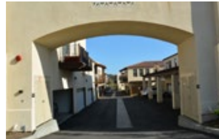
Example of mechanical equipment well-screened by an architectural element incorporated into the building's composition.
