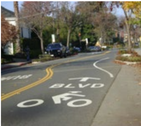
TOP TO BOTTOM —Examples of a Class II separated bike lane and Class III bike route shared with vehicle traffic
