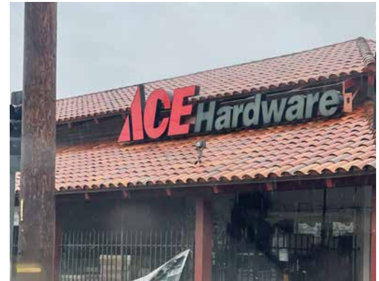
Suite 1056 - ACE - Channel Letters on exposed raceway (1) 4'-0" high x 22'-9" wide
