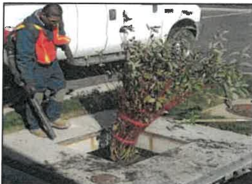
5. Clean area around Filterra
