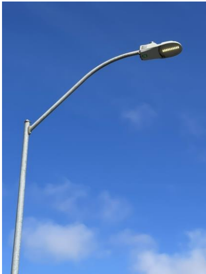
Typical Day Burning Streetlight
