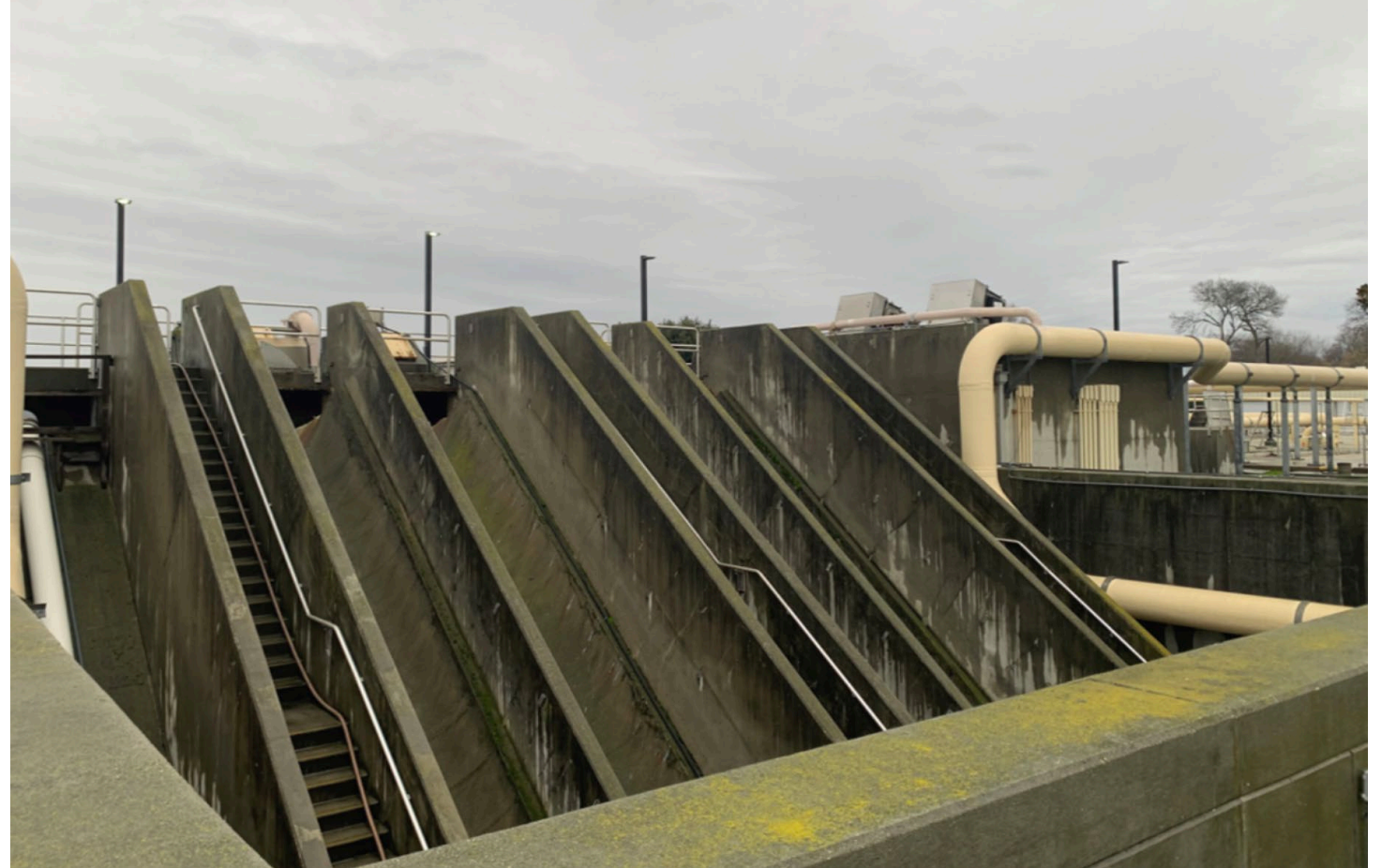
Progress on Water Infrastructure Projects
