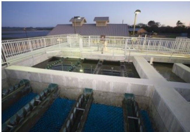
Figure 12: Water Treatment Plant
